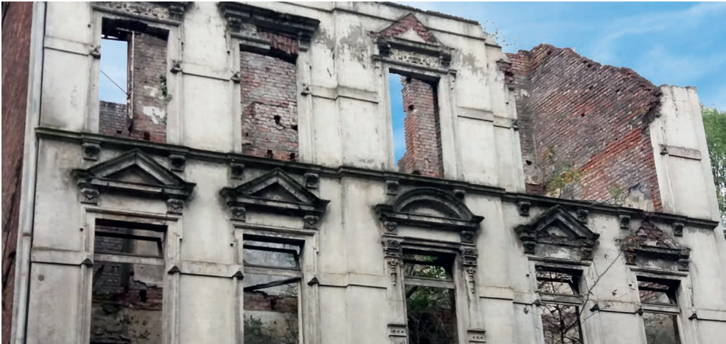
Abb. 19: Problemimmobilie in Wuppertal
